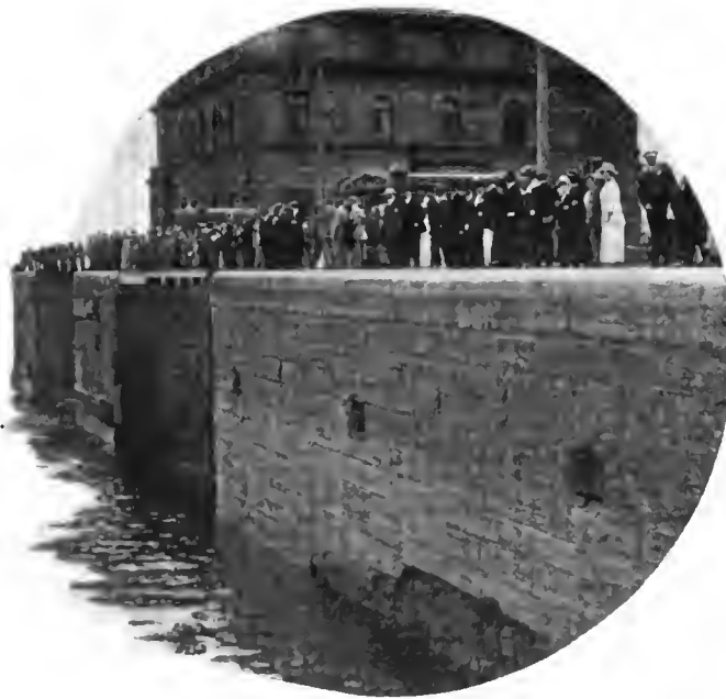
The engineers with friends inspecting the locks at the Soo. The power house for operating the gates is in the background. The semi-crescent shaped recesses in the wall are the gates for the lock, both being open and the water at low level, or empty dock
